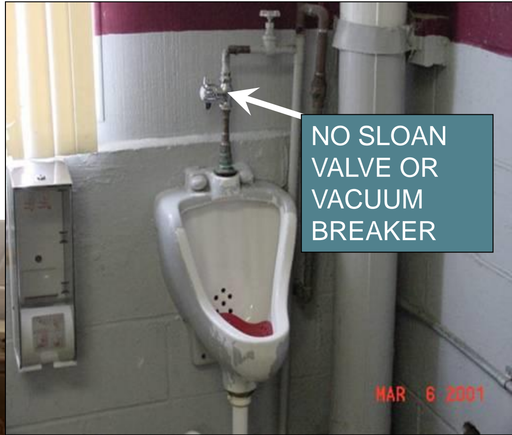
Unapproved Anti-Siphon Valve
