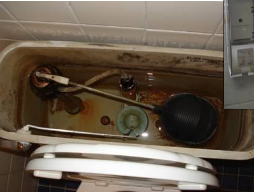
Unapproved Anti-Siphon Valve
